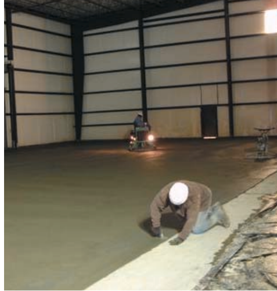
To help eliminate cracking while providing the durability needed, the 8-inch-thick slab floor was created using Grace’s STRUX® 90/40, Eclipse Floor®, and ADVA® 140M.
