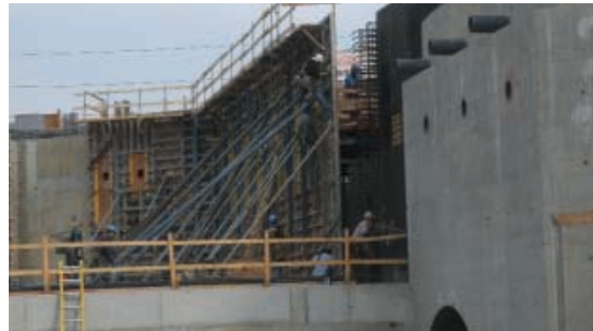
The viewing tanks are among the largest in the world; some are as high as 30' tall and 4' thick at the base.
