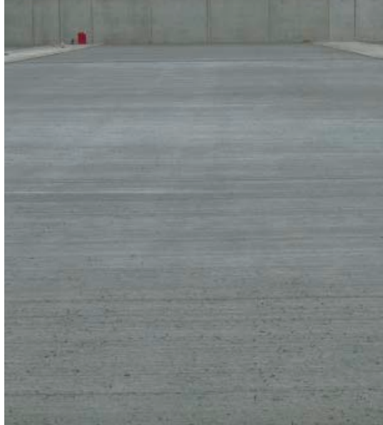
STRUX provided a high performance solution that enabled the job to be completed on time and on budget.
