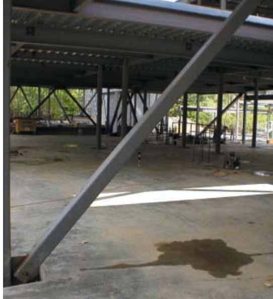
The use of the latest generation of synthetic macro fibers produced a smooth, slick finish quickly and efficiently.
