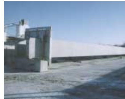
Grace admixtures enhanced the appearance, strength and durability of the guideway foundations and superstructure.
