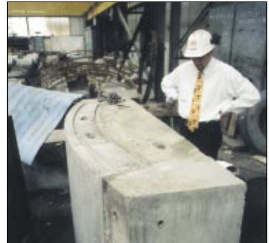
SCC is used to produce precast tunnel segments without vibration.
