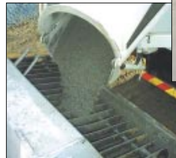
SCC flows and compacts around obstacles and reinforcement to give complete consolidation.
