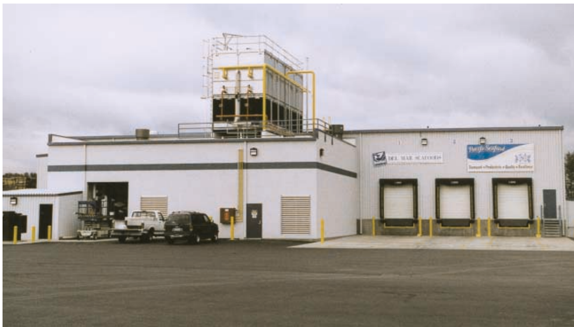
The Columbia Colstor Fish Processing Plant Woodland, Washington, USA
