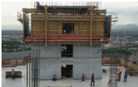
Using SCC with ADVA® 408 increased the concrete's compressive strength to over 13,000 psi, and improved consistency as well as slump retention.
